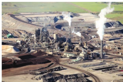
Mines and construction sites
