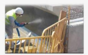
Water industry, for storage tanks and pipeline corrosion protection.
